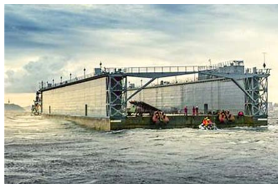
Reinforced concrete floating dock, outer side mooring beam, protected by PPM from the action of salt fog and seawater
