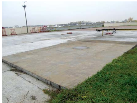
Concrete aircraft sludge parking, protected by polyfunctional polyurethane material (PPM)
