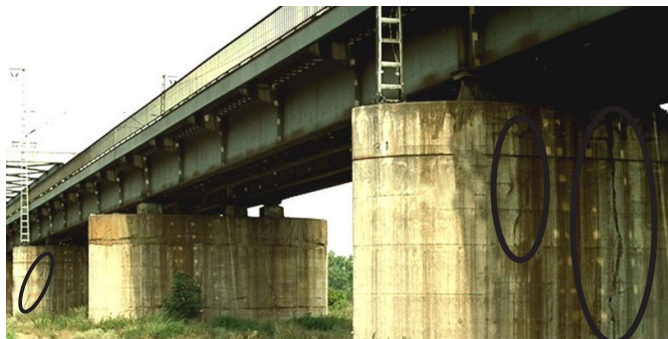
General appearance of pillars of the bridge, damaged by cracks
