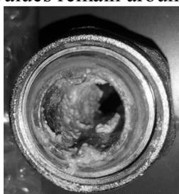
Fig. 1. Photograph of the inside of a cooling convector in a new building
